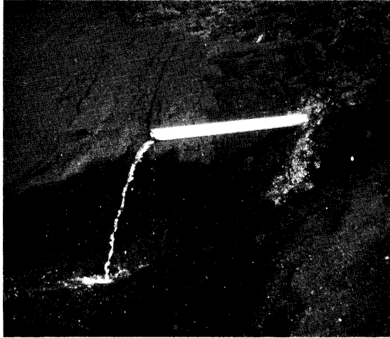
Figure 11. Horizontal drain 250 meters long to reduce pore water pressure in the slope at a major coal mine.
